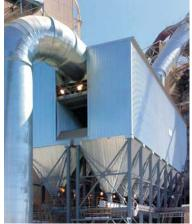
Mikro-Pulsaire® Pulse-Jet Collector. MikroPul invented the pulse-jet and continued innovations, such as our patented inlets, keep the Mikro-Pusaire at the forefront in operating performance and value.
