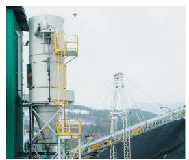
RAF-IS Reverse Air Collector for Hazardous Dust. All electrical components are located outside the housing and no outside oxygen is introduced. These and many other features make the RAF-IS the world's safest dust collector. Ideal for PRB coal and other volatile particulate.
