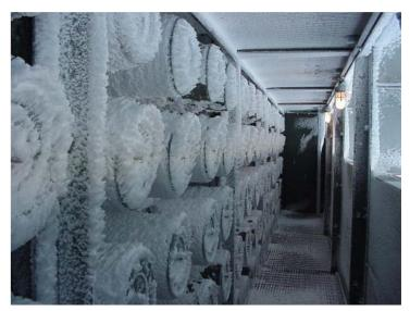
Regardless of your style of filter house, self-cleaning Pulse or barrier style static system, frost, ice and snow can quickly load onto your filers and impact your airflow and choking off needed airflow to your turbine.
